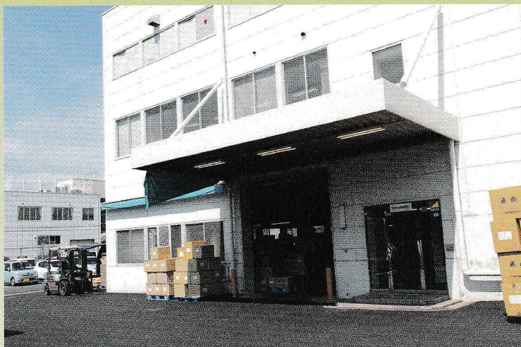
本社社屋 HEAD QUARTOR & PLANT
